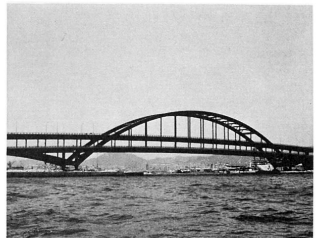
KOBE OHASHI BRIDGE (KOBE CITY)
