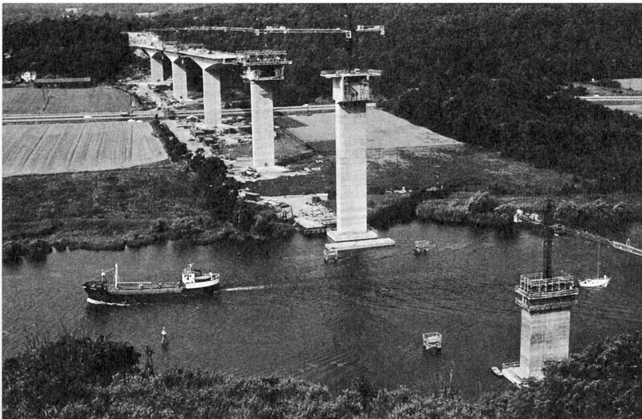
Fig. 4 The bridge under construction
