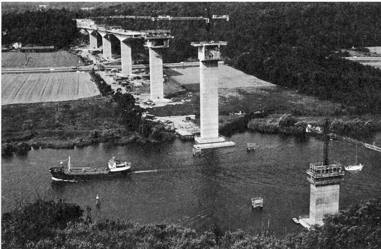
Fig. 4 The bridge under construction
