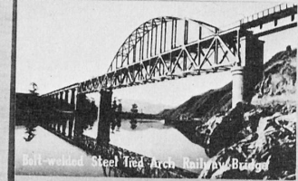
Laju Bridge. Southwest China. built in 1967. Span 112m.
