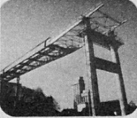
Sennett (single bridge) 3 spans: 51 + 62 + 71 + 83 + 8 + 50 + 36 = 654 m steel weight: 1,220 t recast concrete slab: 13,890 m 3
