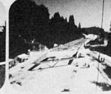
Seyon (single bridge) 2 spans: 30.8 + 59.3 = 90.1 m steel weight: 381 t launched concrete slab: 1,960 m 3
