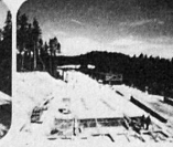
Chaudeland (twin bridge) 5 spans: 44 + 54 + 54 + 51 + 41 = 244 m steel weight: 646 t launched concrete slab: 6,440 m 3
