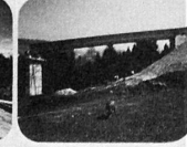
Louvauch (single bridge) 4 spans: 52 + 65 + 52 + 52 = 221 m steel weight: 260 t cast in place concrete slab: 2,260 m 3
