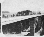
Gilwe (twin bridge) 3 spans: 56 + 71 + 56 = 183 m steel weight: 520 t precast concrete slab: 4,100 m 3
