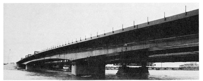
A grillage comprising 40 drilled piles, each 17 m long with a diameter of 1.2 m, was made for the river piers. At river bed level the piles were joined by means of a reinforced concrete slab. An apron made of sheet pile wall planks was sunk down to a depth of 8.5 m to counteract floodwater pit formation and erosion. The reinforced concrete river pier was built upon this base structure and protected against erosion from sediment transport by a specially wear-resistant facing layer.
