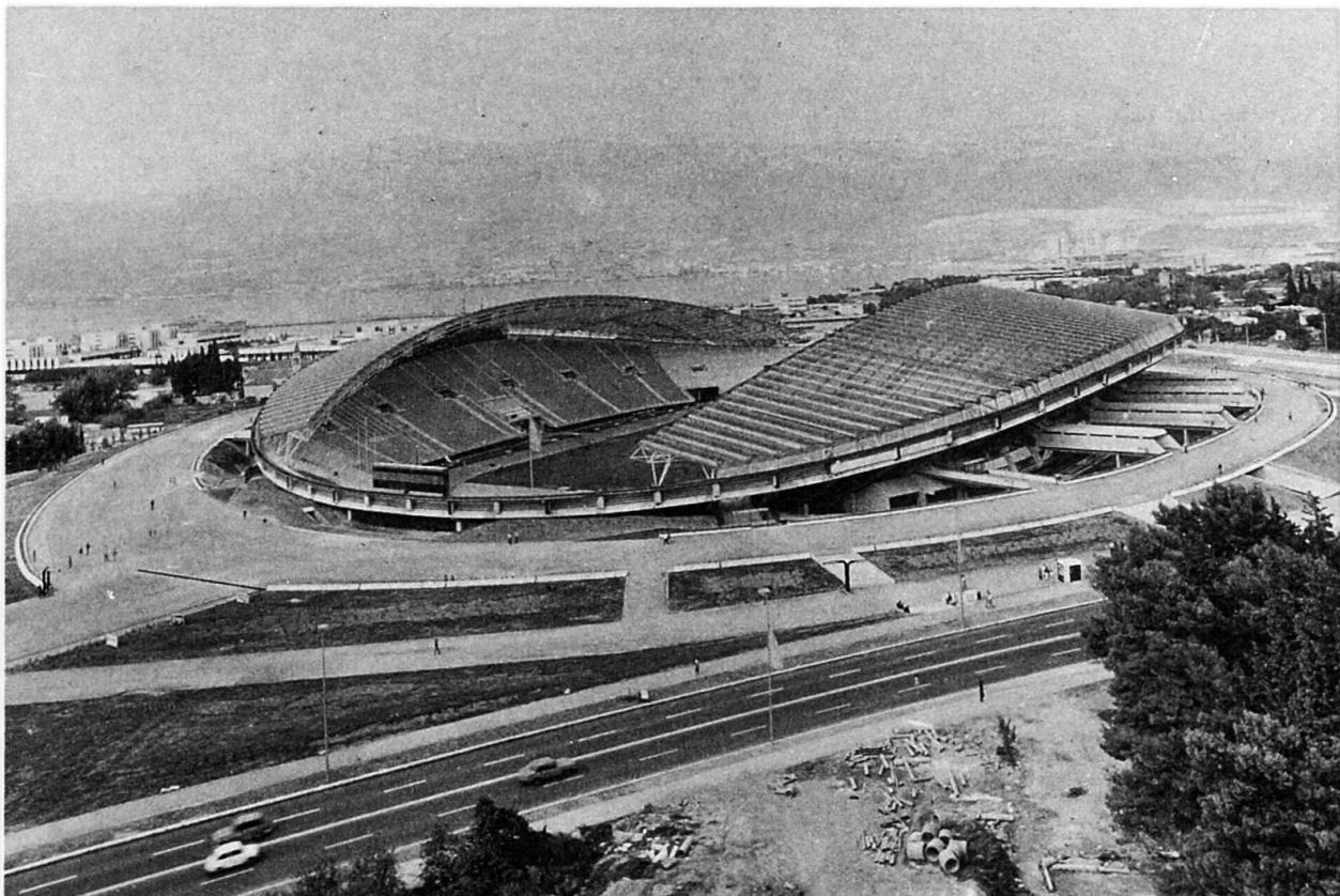
Fig. 1 View to the City Stadium
