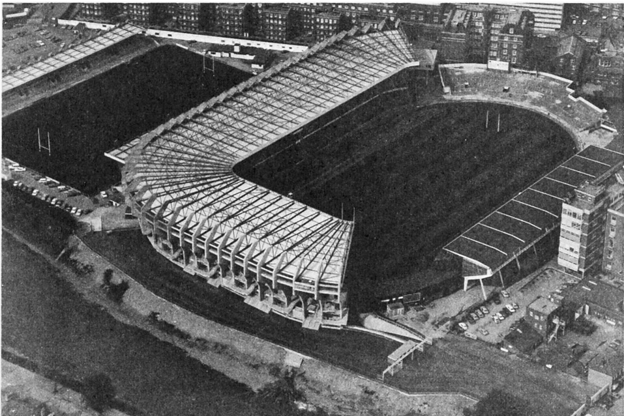
Aerial photograph of the Stadium taken in 1978
