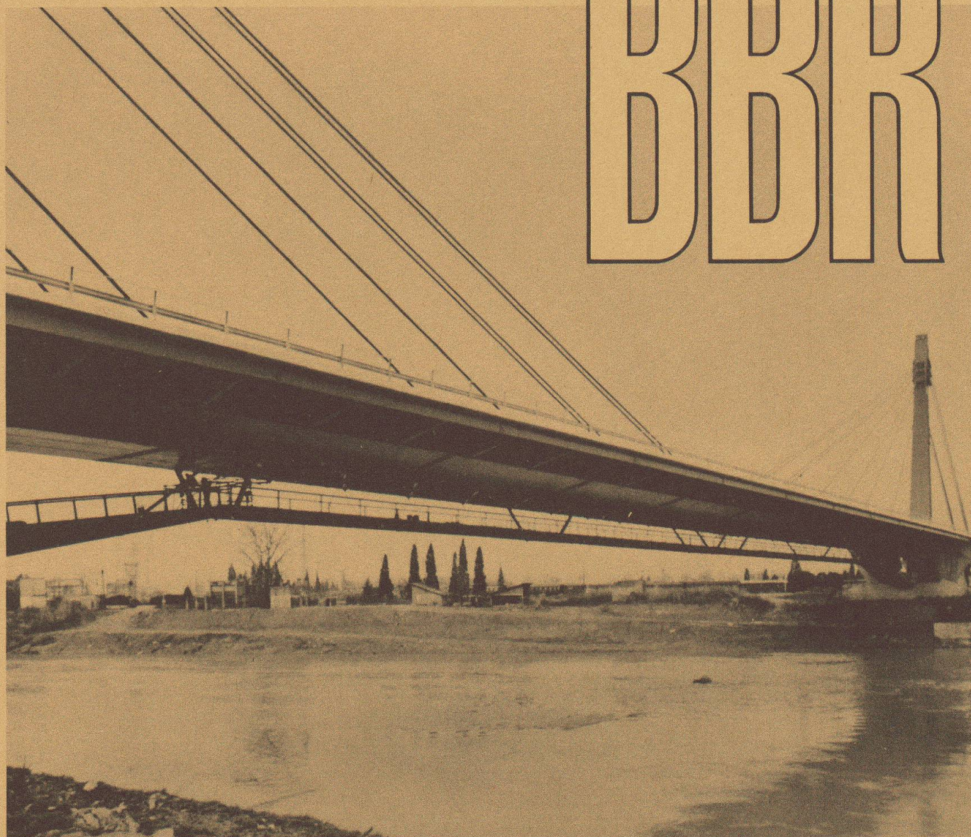
BBRV-HiAm stay-cables for highway bridge over the river Arno near Florence, Italy
