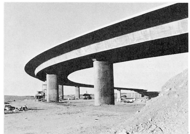
Fig. 2 Nearly completed interchange bridge, before mounting the precast parapet elements
