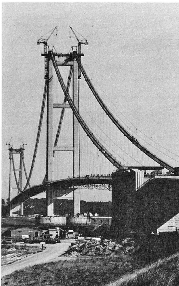
Fig. 4 General view of the structure, October 1980. (Note the effect of lack of asphalt dead load on the continuity of the profile at the tower.)
