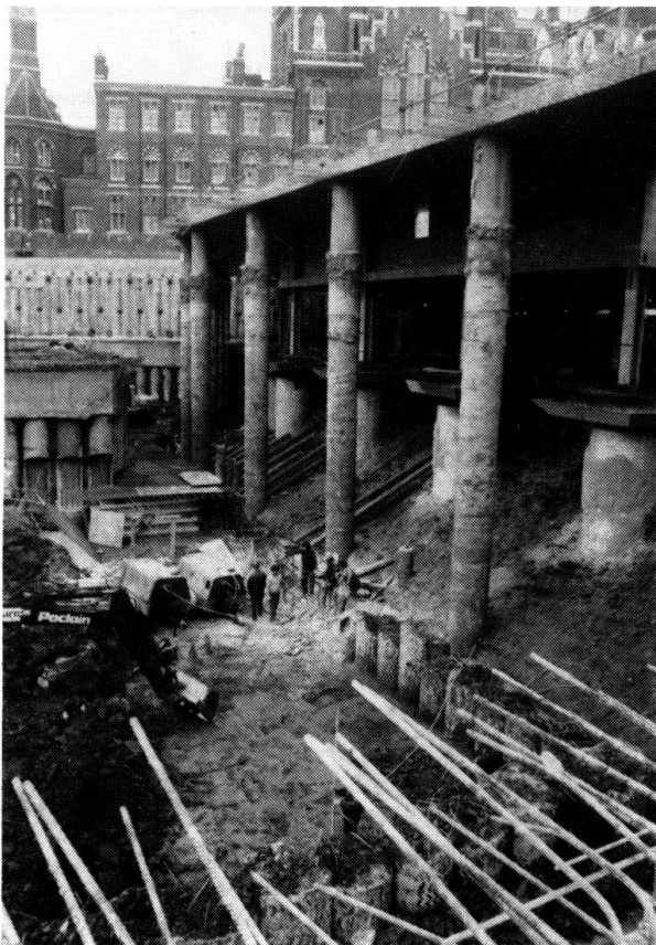
Figure 3 Central area excavation
