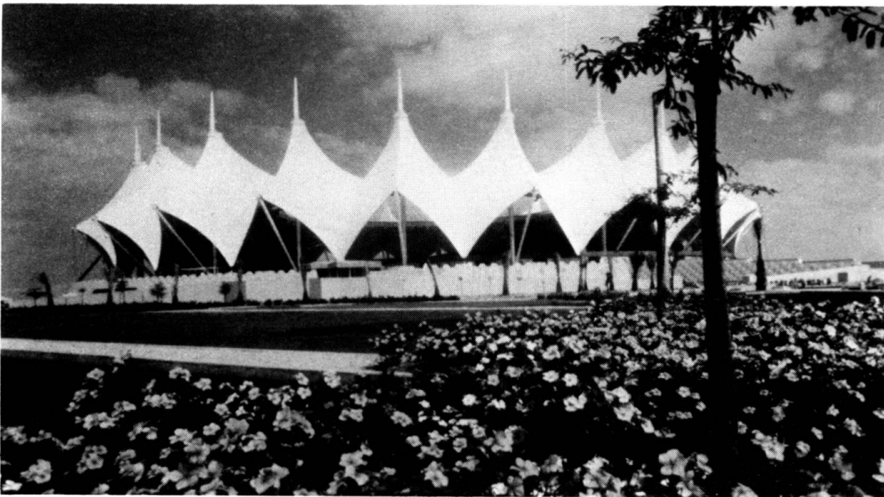
Fig. 7: Roof after Completion
