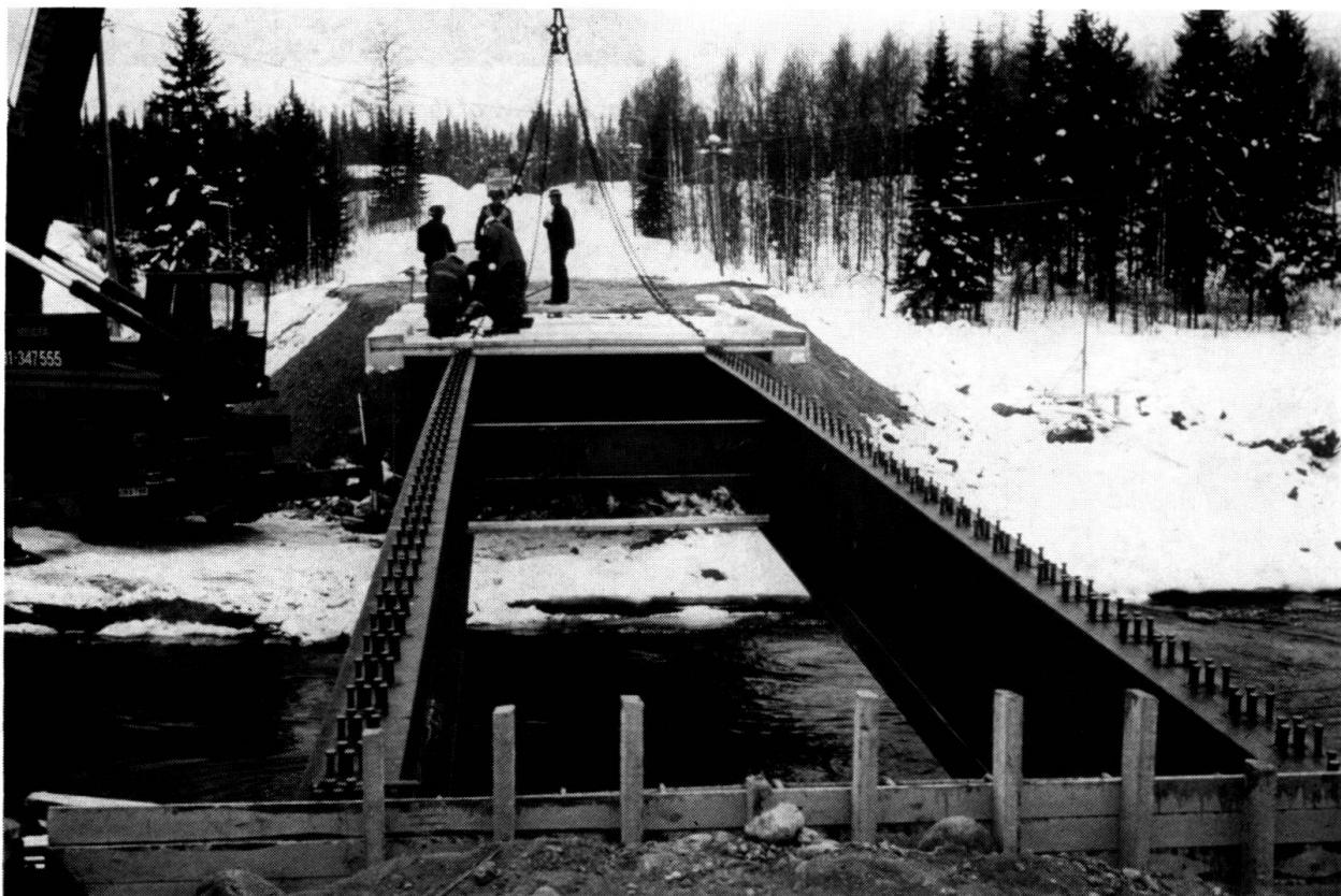
Fig. 3 Assembly in progress
