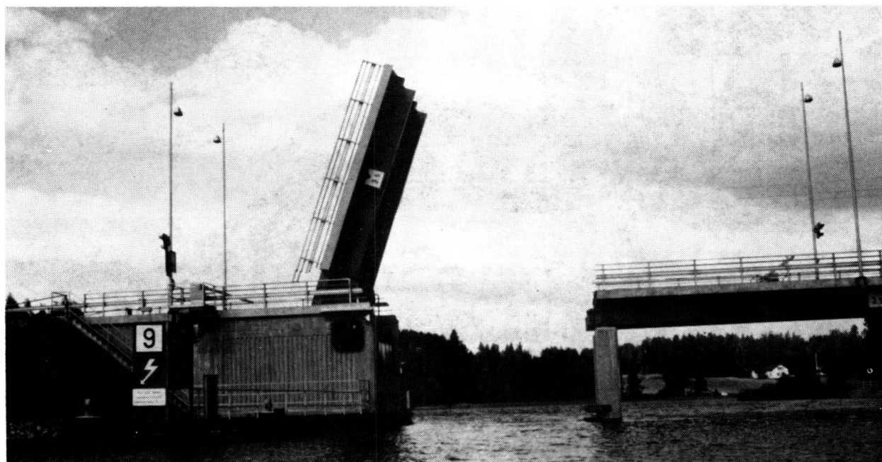
Fig. 1 Bridge in the «open»-position, view from the channel
