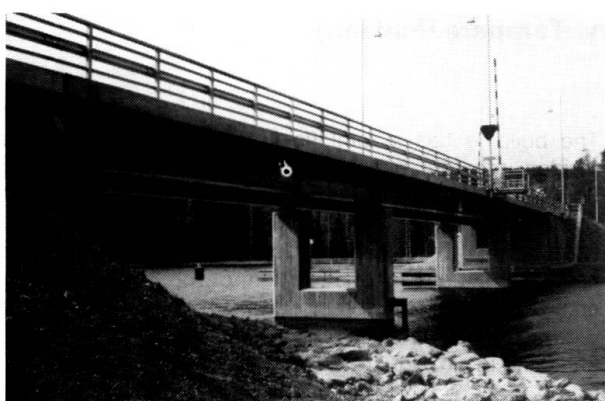
Fig. 3 General view of the bridge
