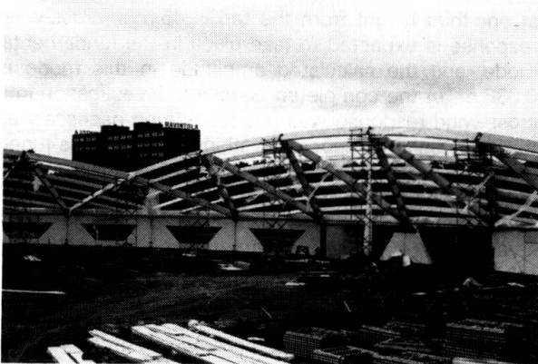
Erection of the dome
