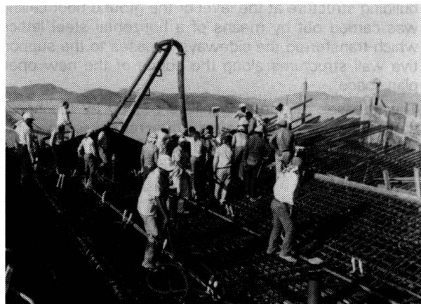
Fig. 4 Concreting of a part of the suspended span
