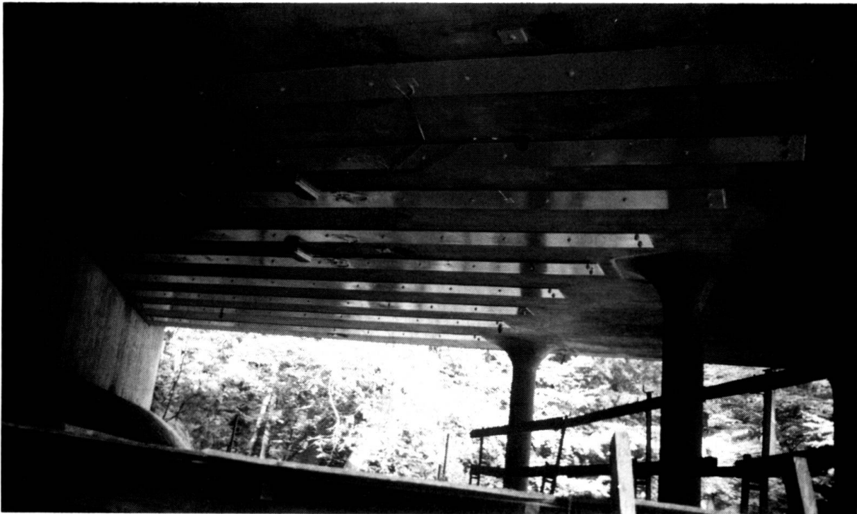
Bridge deck reinforced with bonded steel plates. The strain gauges were used to verify the efficiency of the bonding. The bolts are removed after completion.
