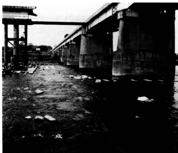
Fig. 3 After repair (Iwaide Bridge)
