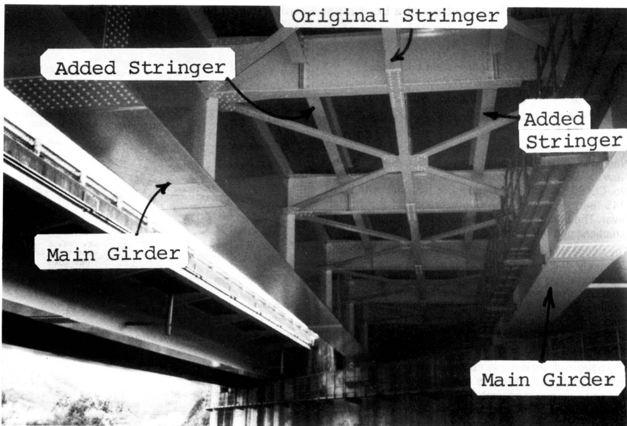
Photo 1 General View of Strengthening
