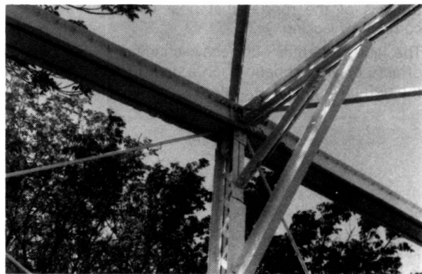
Fig. 5 View of upper chord with new member in place
