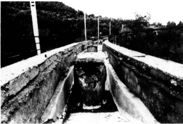
Fig. 2 A view of the inside of viaduct after removing of filling
