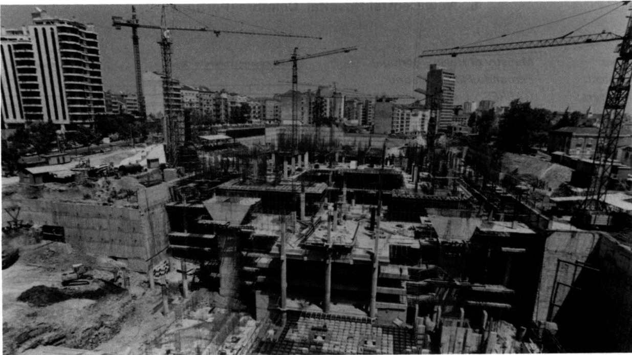
Fig. 2 General view of the site construction
