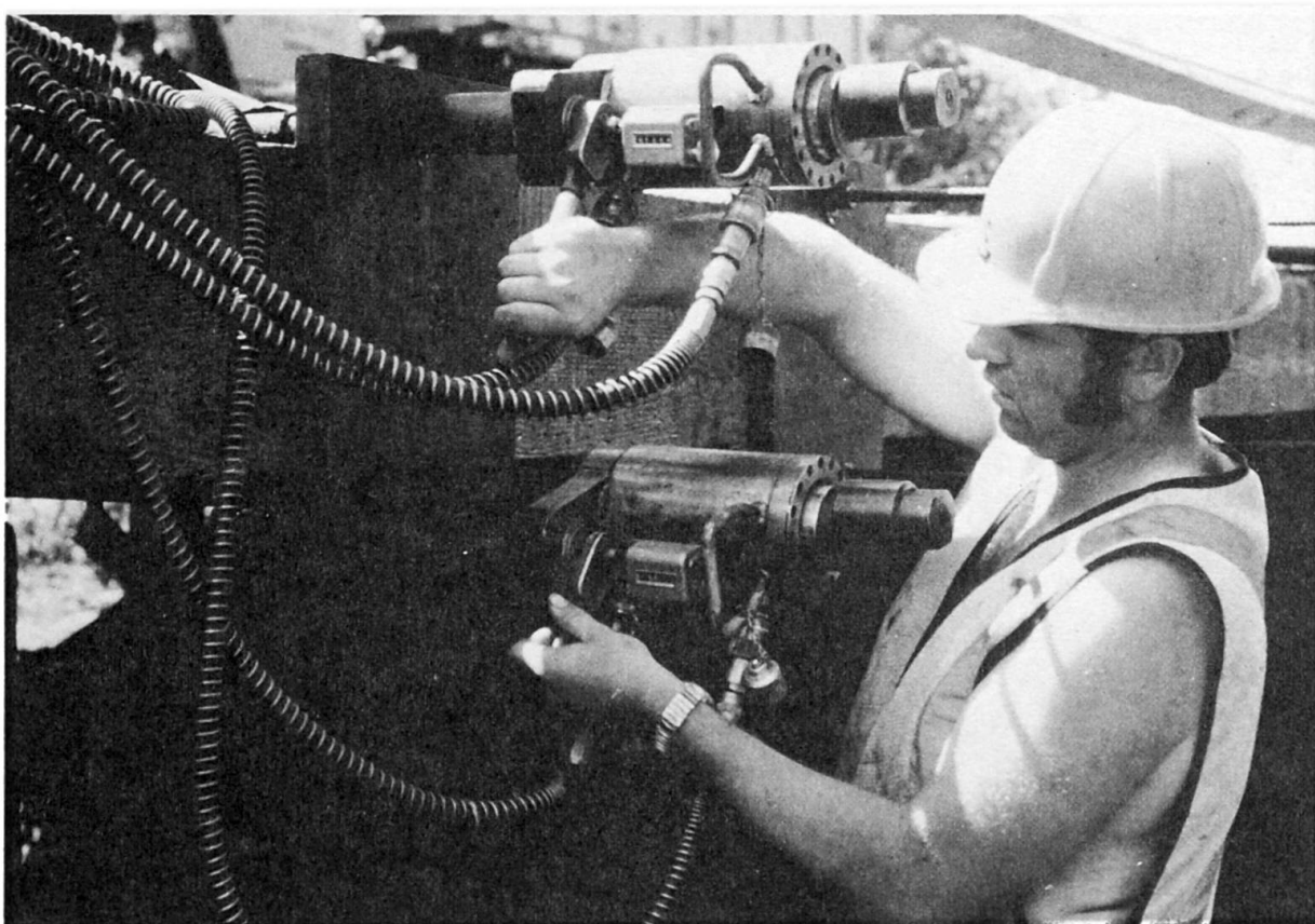
Figure 6 Prestressing of Hebert Creek Bridge
