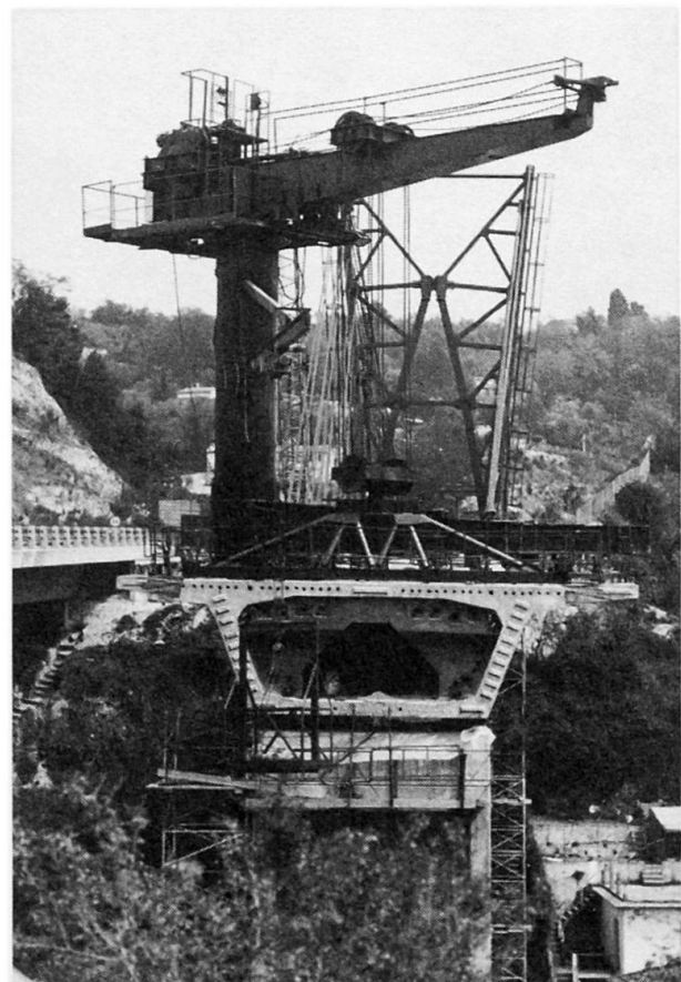
Fig. 2 - The lifting device
