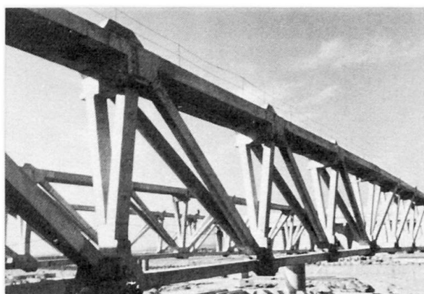
Figures 1 and 2 : Simplified drawing of Tehran stadium truss girder : half-span — cross section — photo
