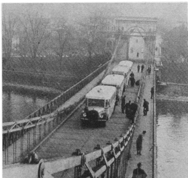
Fig. 1 The Kettenbrücke in Aarau, here during the 1945 static tests. Photograph from [1].
