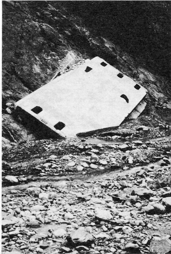
FIG. 2 200 Ton Bridge slab after the flash flood.
