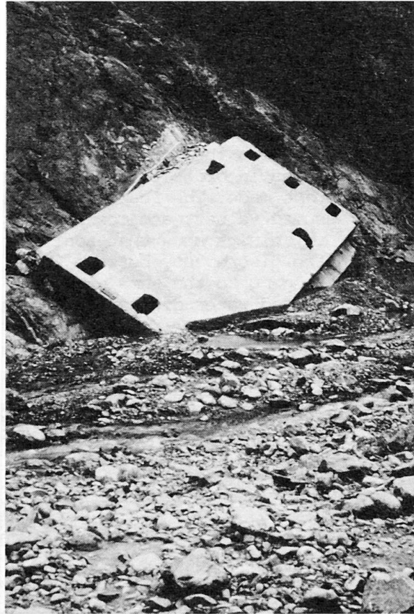
FIG. 2 200 Ton Bridge slab after the flash flood.
