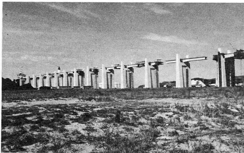
Fig. 18 Construction of Bannosu Viaduct
