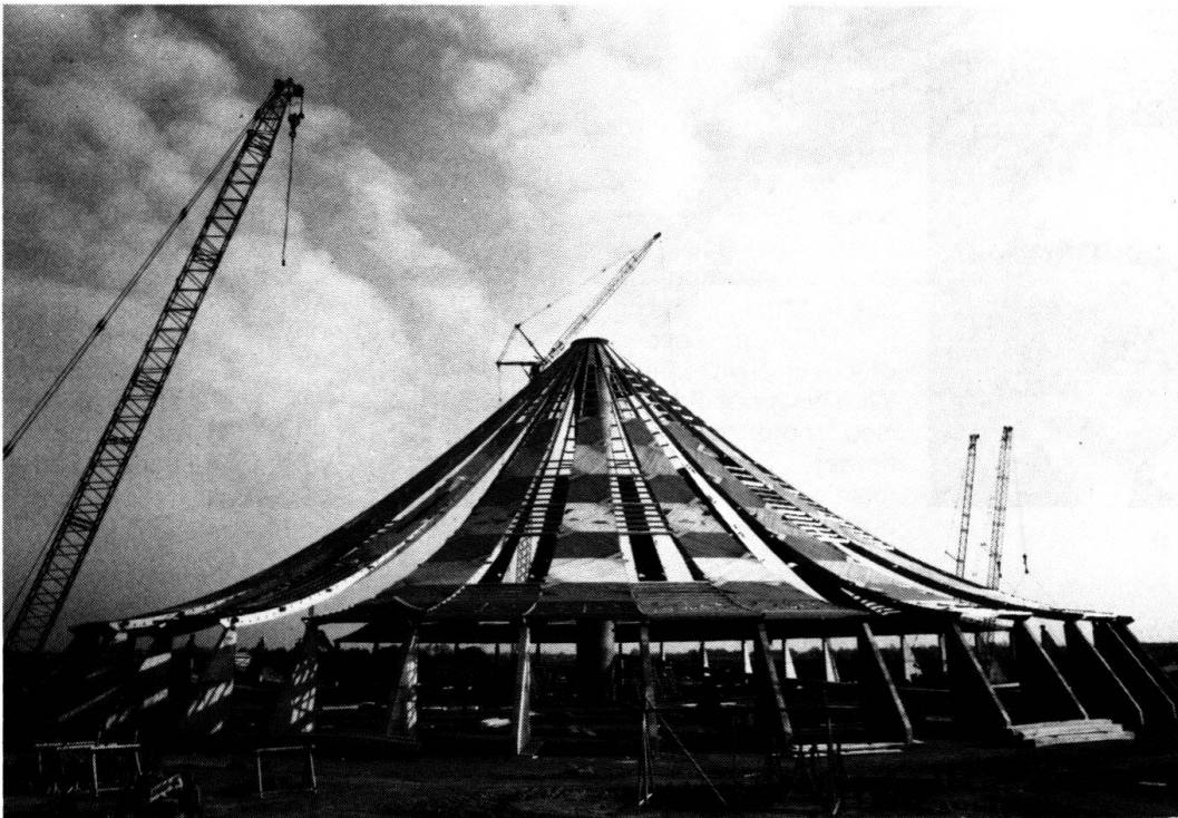
Fig. 1 : The hanging timber shell in Vienna during construction.
