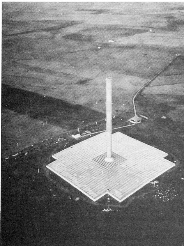
Fig. 2: Aerial photograph of the experimental facility at Manzanares, Spain (height of chimney 200 m; chimney radius 5 m; collector 120 m/120 m; rotor diameter 10 m; nominal speed 100 rpm)
