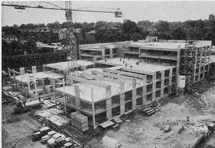
Fig. 15 - Multi-storey car park, Croydon.
