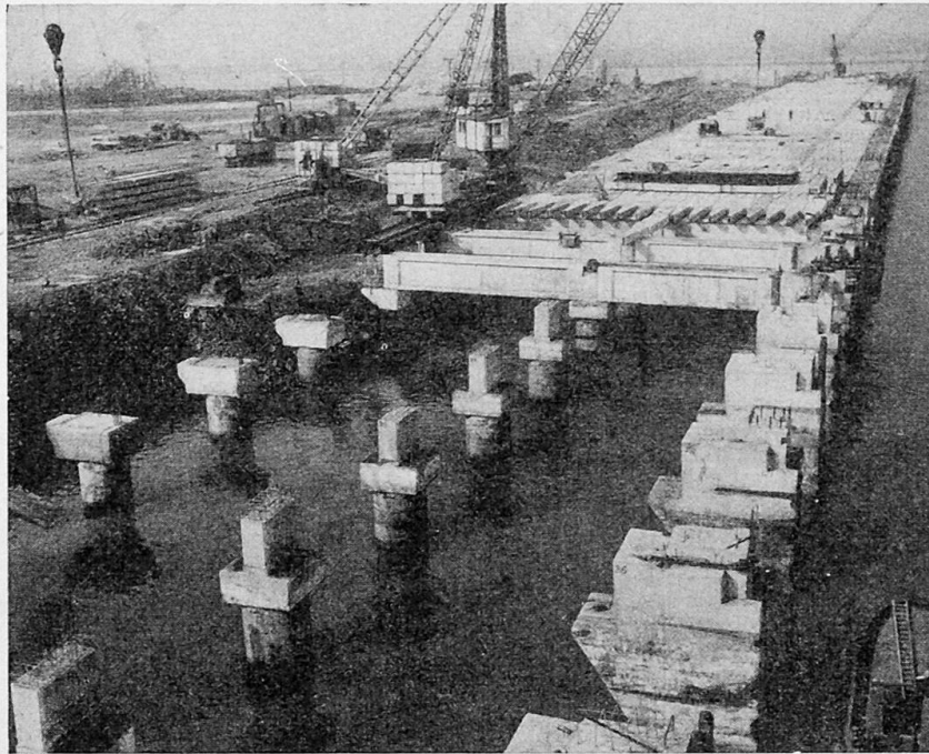
Fig. 14 - Tees Dock Quay of precast concrete elements manufactured on site.
