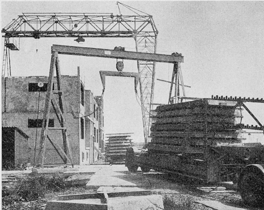
Fig. 4.2 - The Rottinghuis-housing system. The lorries with the floor elements are unloaded from the trailer by a fixed crane. In the background the portal framed crane for mounting the elements.
