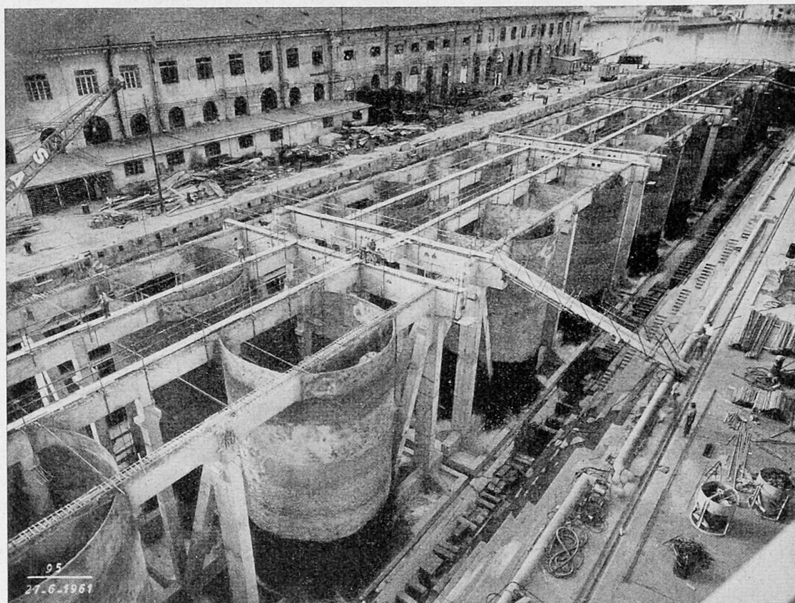
Fig. 13 - Edisonvolta thermal power plant, La Spezia. In-situ prefabrication of the fuel discharging wharf (Impresa SALCI).
