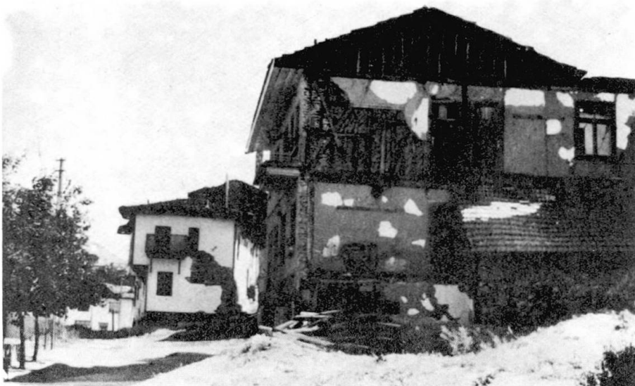
Figure 4. Typical Wood Frame Structure (Hımsı)
