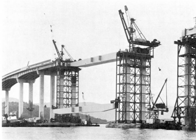
Fig. 11 Box girder erection
