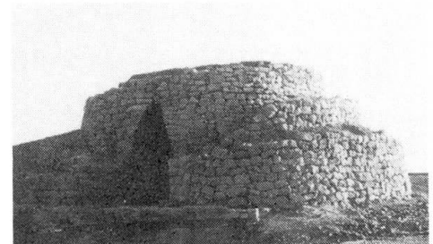
Fig 2 Corbelled arch
