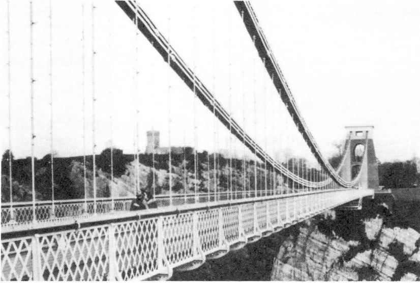
Fig.7 Clifton Bridge. © Author
