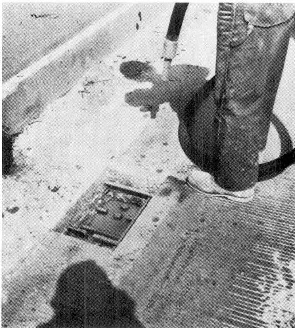
Fig. 11 Portion of Slab Removed to Gain Access to Flange
