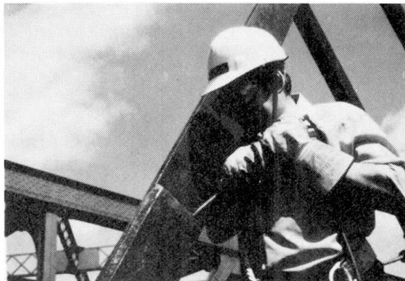
Figure 19 Peening welds
