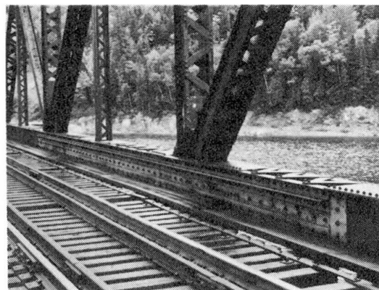
Figure 12 Member spliced
