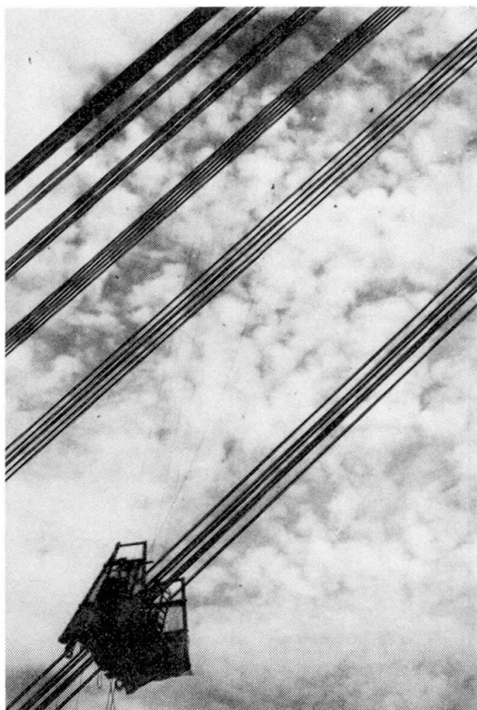
Fig. 10 Inspection of Cables
