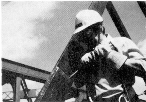
Figure 19 Peening welds
