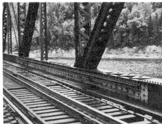
Figure 12 Member spliced
