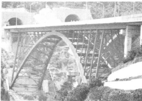
Fig.2 An arch bridge that caused lateral vibration.
