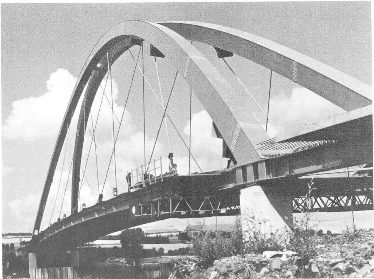
Fig. 10 Bridge at Hermalle.
