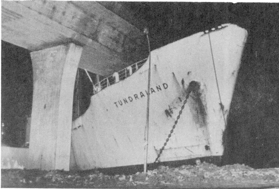
Fig. 8 Drammen Bridge; Nearly catastrophe
