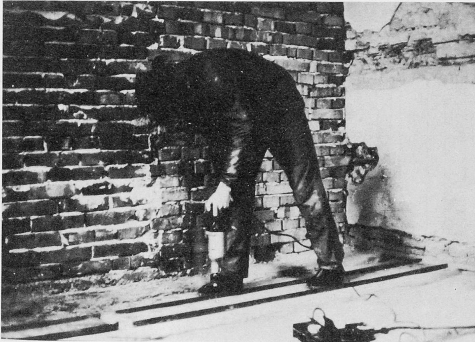
Fig. 6. Rough drilling with a drilling template
