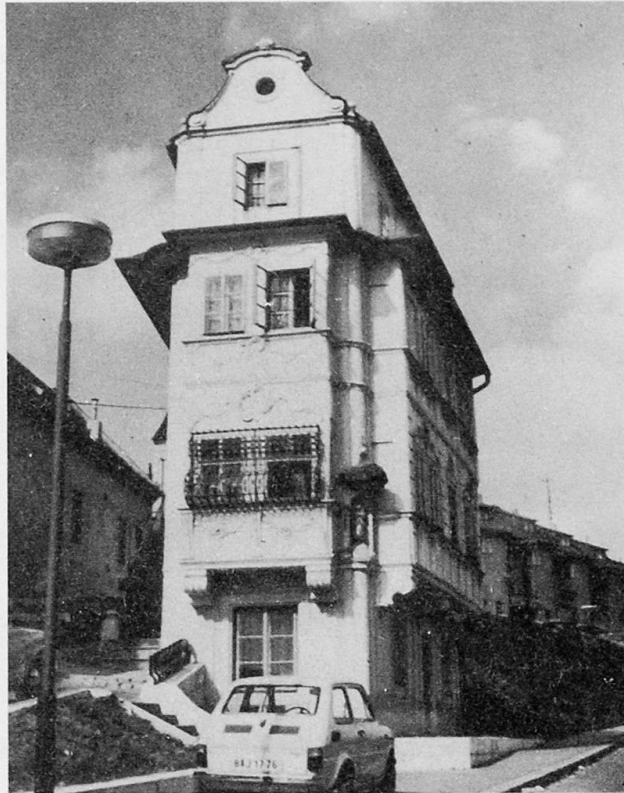
Fig. 5. The house "The GOOD SHEPHERD" in Bratislava with strengthened ceilings from 1960.
