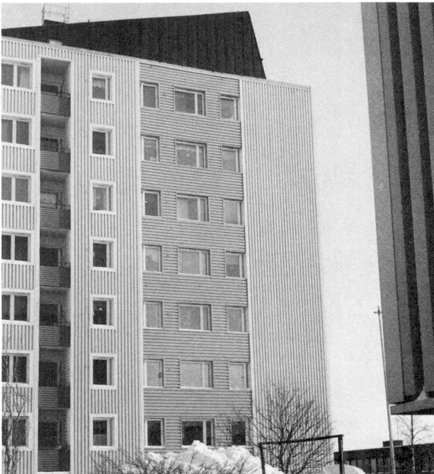
Fig. 3 High-rise-buildings are simple to renovate with steel sheet
