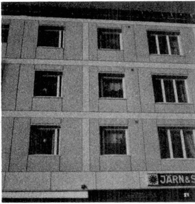
Fig. 6 Steel sheet units are similar to rendering
