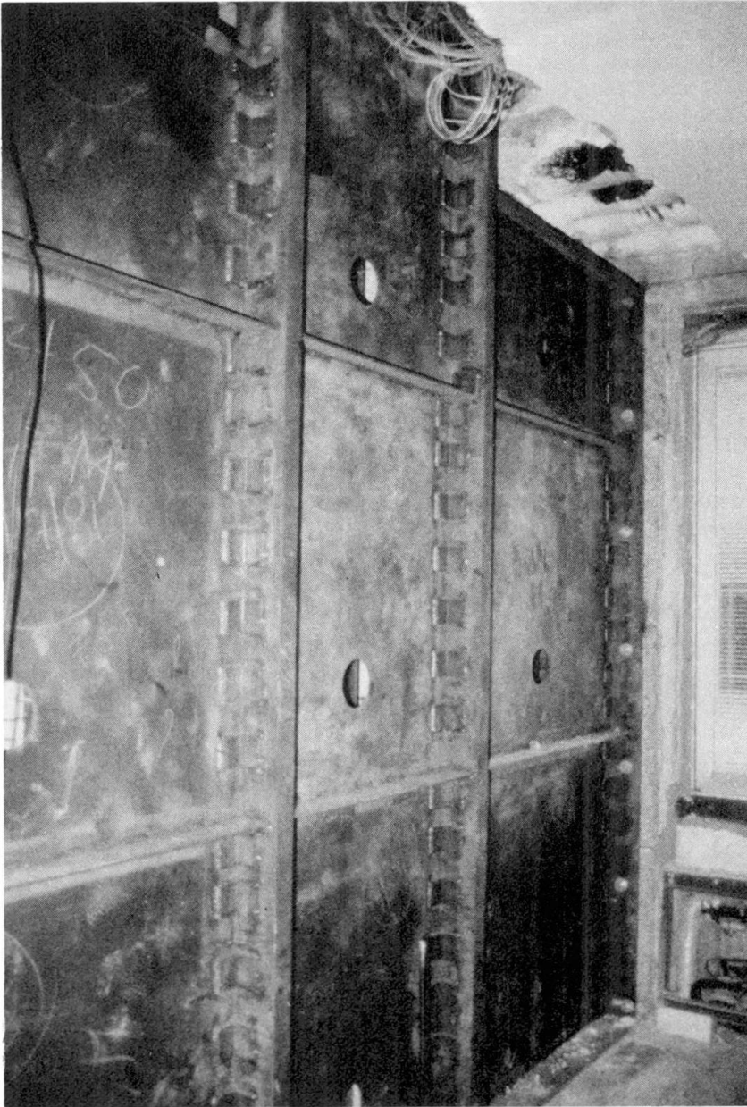
Fig. 4 Steel Plate Shear Wall
