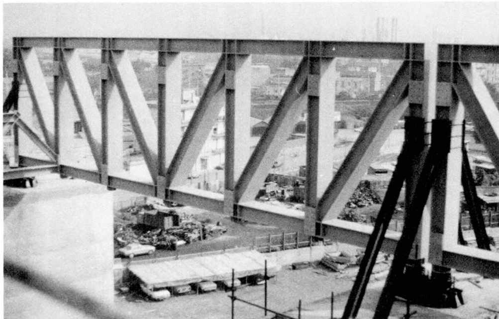
Fig. 3 - Longitudinal reticular girder erected on the top of the concrete towers.
