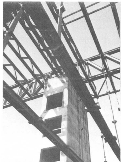
Fig. 5 - Ties and floor beams hanged to the top grid.
