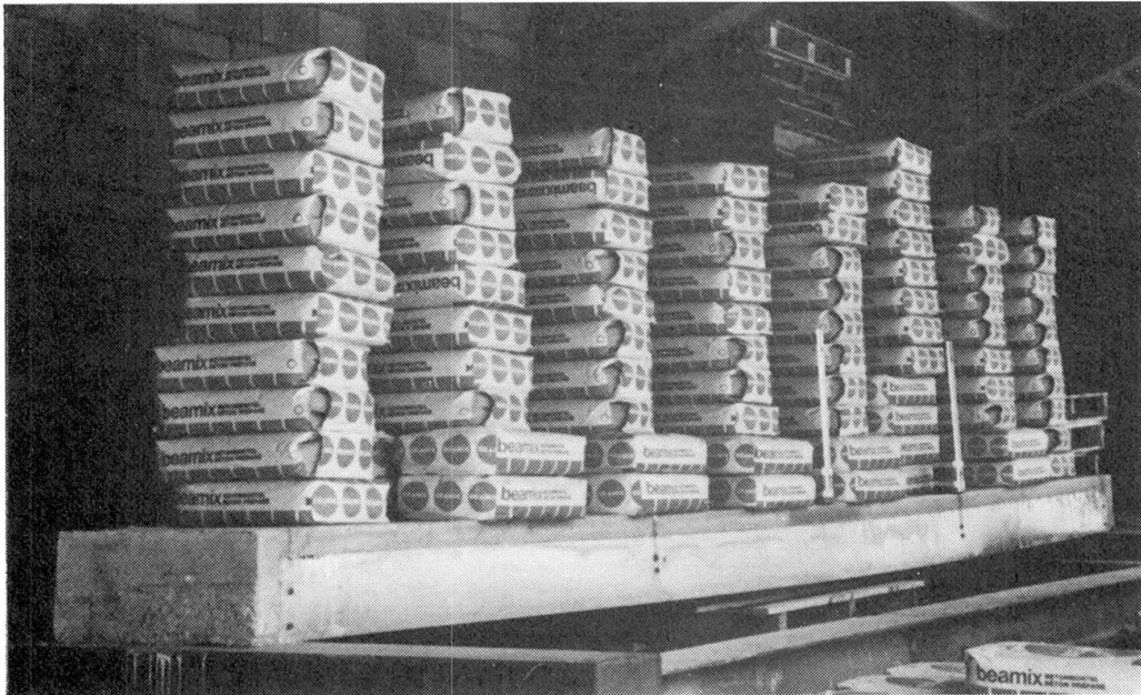
Fig. 11 Composite deck element under test loading (field test)
