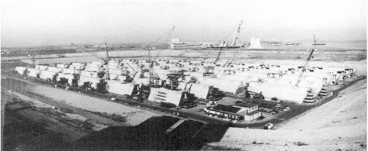
Photo 2 Sill-beams in construction dock (Jan. '85)
